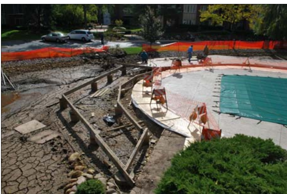
Ponds emptied & deck removed
