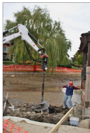
Drilling new holes.
