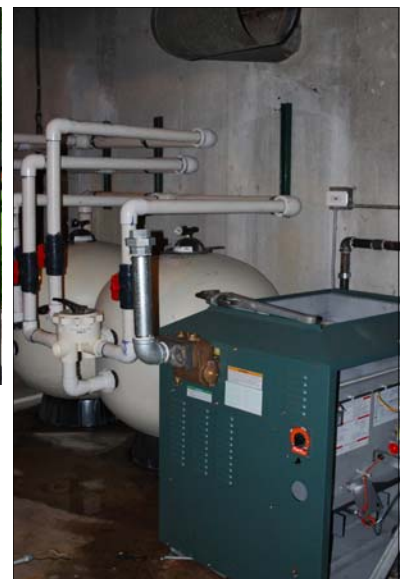
Right: In with the new, smaller high-efficiency pool heater!
